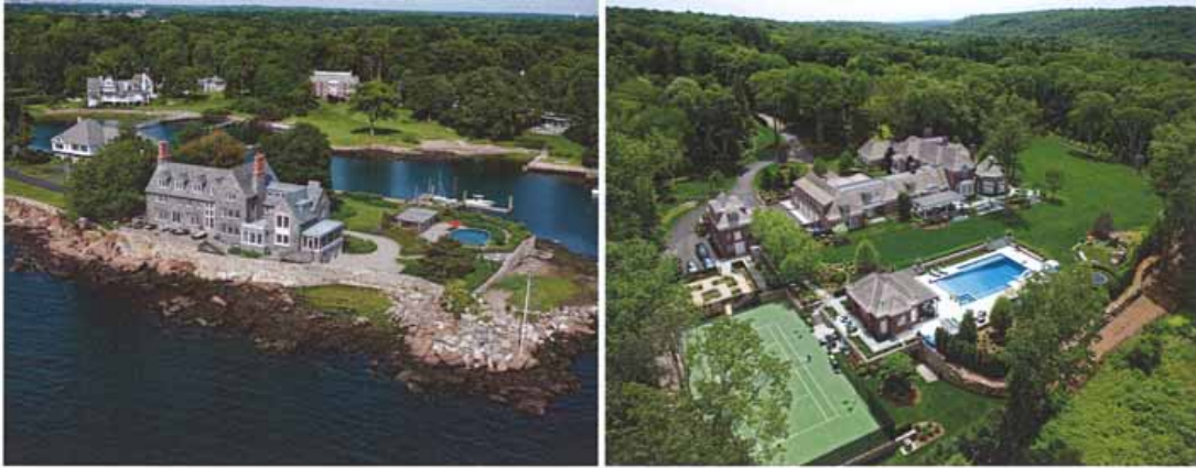
ABOVE: Taconic was selected as the builder for these Suburban Luxury Projects: (From the left) 14,000 sq. ft. Stone House Estate situated on Long Island Sound and Country Estate in Weston, CT
